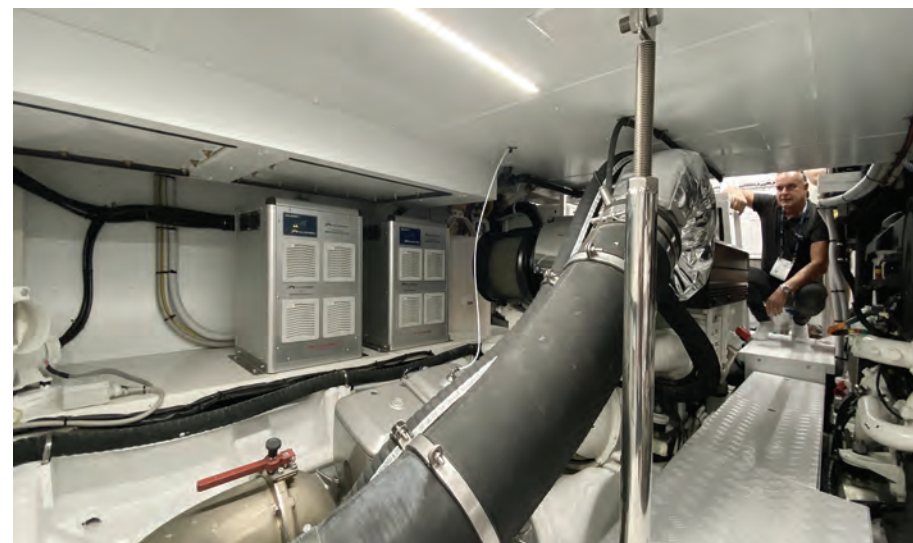
ANG ISO-BOOST 2x25kW installed on a Sanlorenzo Yachts SX88
